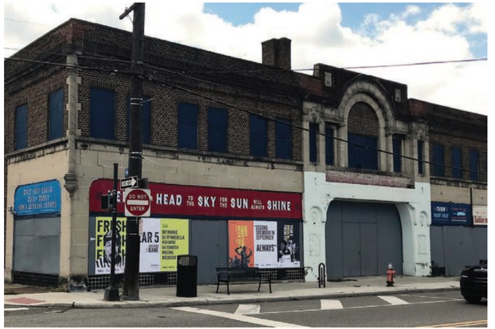
The vacant Moreland Theater Building at the corner of Buckeye Road and East 119th Street may become the cornerstone of an arts district centered on Black creators and entrepreneurs.
