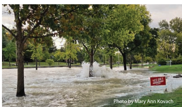
A water main break between 5 and 9 p.m. Oct. 14 flooded the eastbound side of Van Aken Boulevard between Southington and Onaway roads in Shaker Heights. A boil alert was in place until the next evening, and RTA's Blue Line was closed temporarily.
