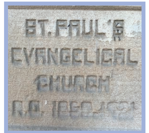
This cornerstone on Batuqui's new Larchmere location reveals some of the building's history.
